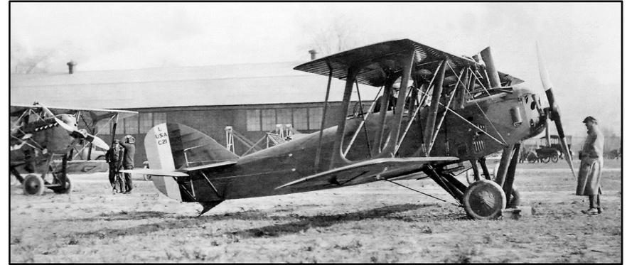
*The LUSAC-21: perhaps the only King-Bugatti-powered aircraft to fly. Note the vertical exhaust stack in front of the upper wing. The nose of a Liberty-powered LUSAC-11 can be seen in the background at left. Although not apparent in this image, the two aircraft were very similar.*
