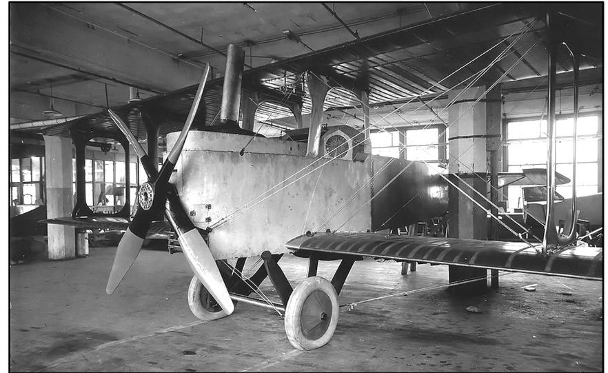
*The King-Bugatti-powered LUSAGH-11 under construction at the Packard factory in Detroit, Michigan at the end of August 1918. Note the exhaust manifold combining the 16 individual exhaust stacks into one vertical pipe and the radiator below the propeller shaft. This aircraft was never completed.*
